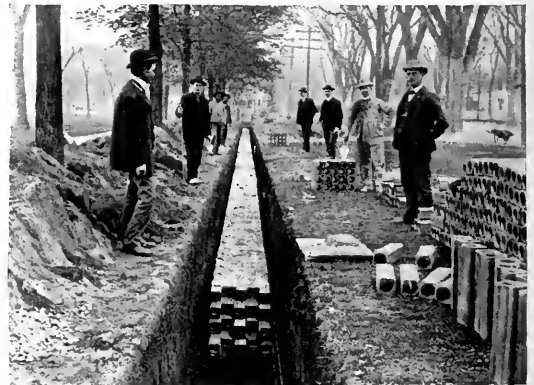
FIG. 2.—UNDERGROUND CONDUITS, SPRINGFIELD, MASS.
